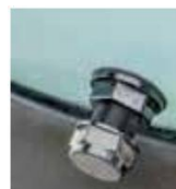
Drenaža filtera Filter drainage
