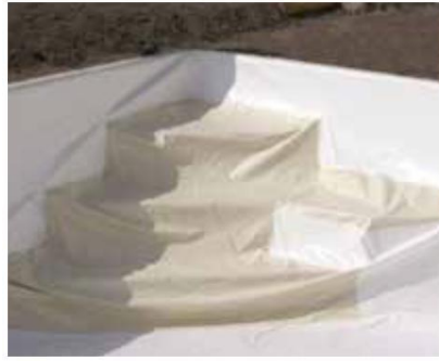
Ugaone stepenice postavljeni liner - Corner stairs laying of the liner
